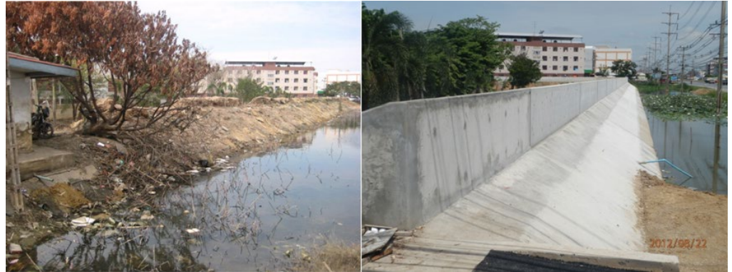
Flood defenses: before and after 2011 flood
